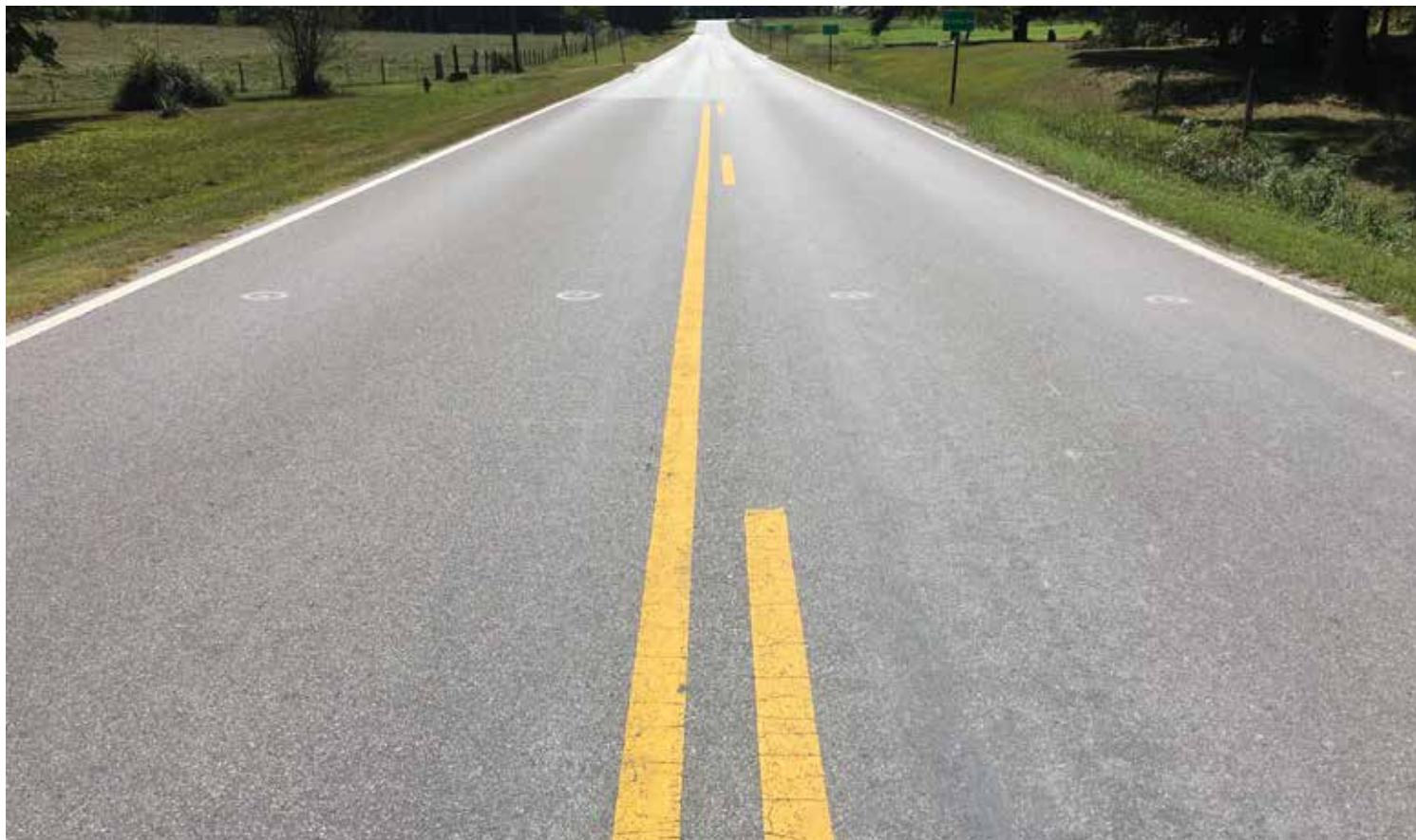
Overall condition of scrub cape seal on Lee Road 159.
