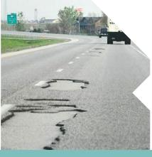
SHOVING AND DELAMINATION CAN OCCUR WHEN BOND COAT IS NOT APPLIED PROPERLY OR WHEN NOT ENOUGH IS USED
